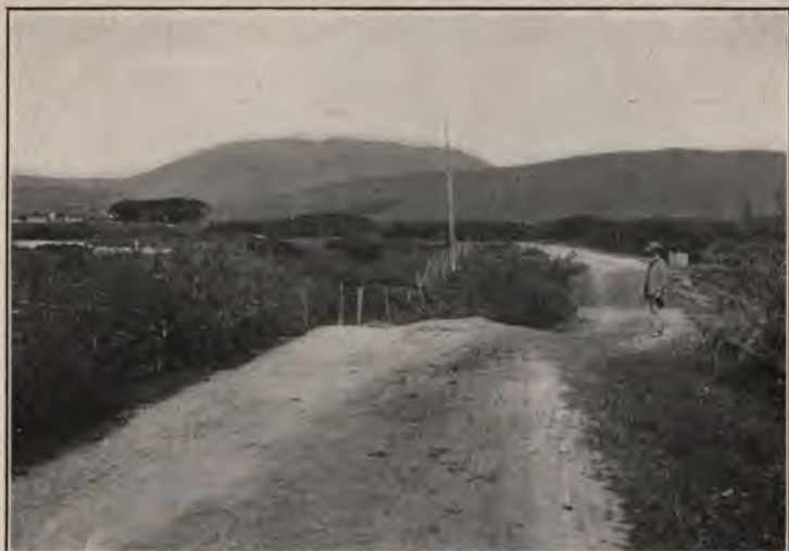
A. Road displaced laterally about twelve feet on line of the great rift near the head of Tomales Bay.
